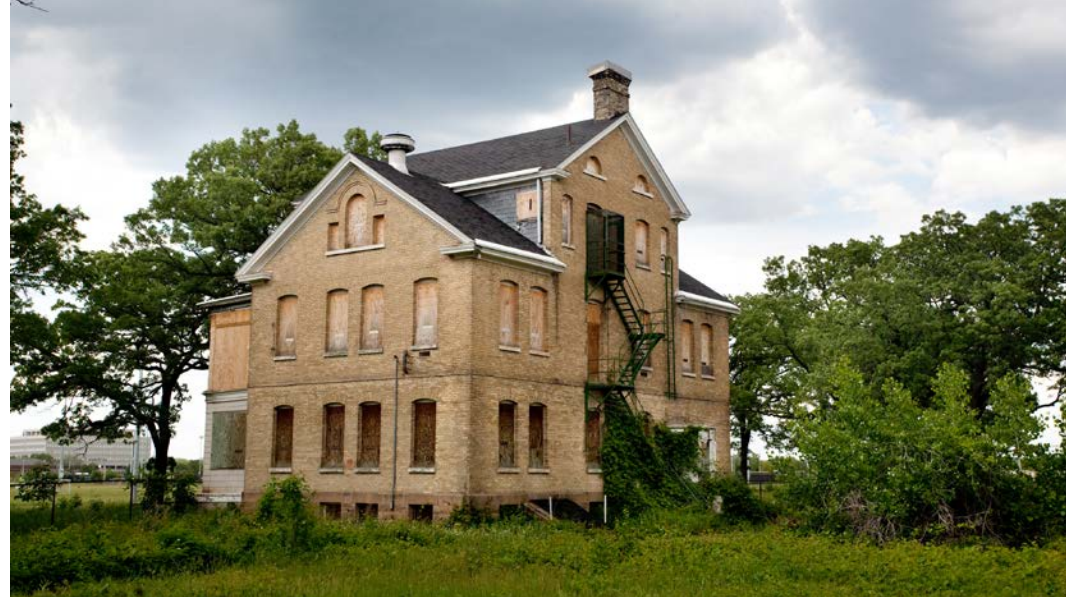
The Band Barracks is one of 26 buildings that are being rehabilitated for low-income housing as part of the project. It has been largely abandoned since the 1970s.
